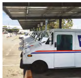
Left: A carport canopy with solar panels has the added benefit of lowering temperatures underneath by as much as 7 degrees compared with the open air.
