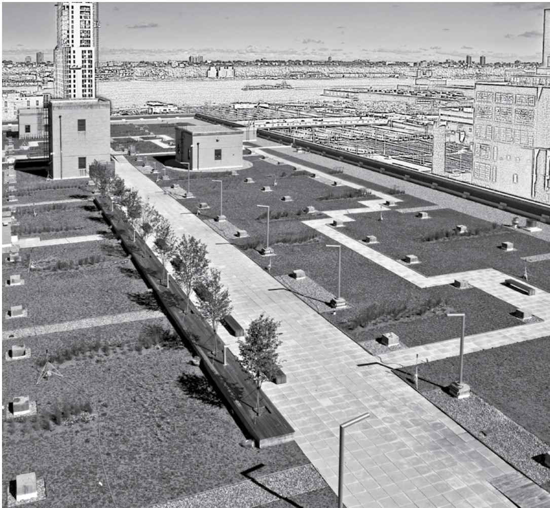
The Green Roof at the Morgan processing facility is the first developed by the Postal Service, and at 109,000 square feet – nearly 2.5 acres – is the largest in New York and one of the largest in the country.
