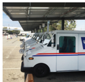
Left: A carport canopy with solar panels has the added benefit of lowering temperatures underneath by as much as 7 degrees compared with the open air.
