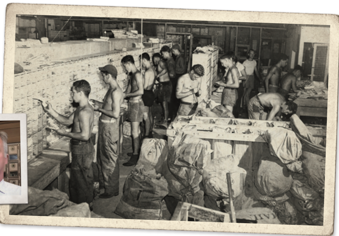
Mail processing in a Quonset hut in the Pacific during World War II
