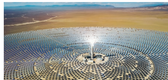
Above: The Crescent Dunes Solar Energy Project, north of Tonopah.
